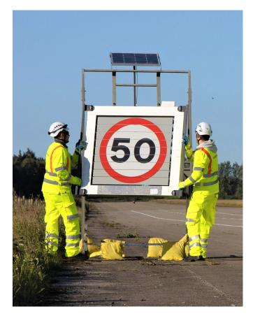
Dynamic Speed Signs have changed this. Using digital technology, the new signs can automatically change to display 40, 50 or 60 mph according to the works programme. This removes the need for operatives to physically change signs which keeps them safe. It also allows traffic to flow freely at 60 mph when works are stopped, minimising disruptions and improving journey times.
